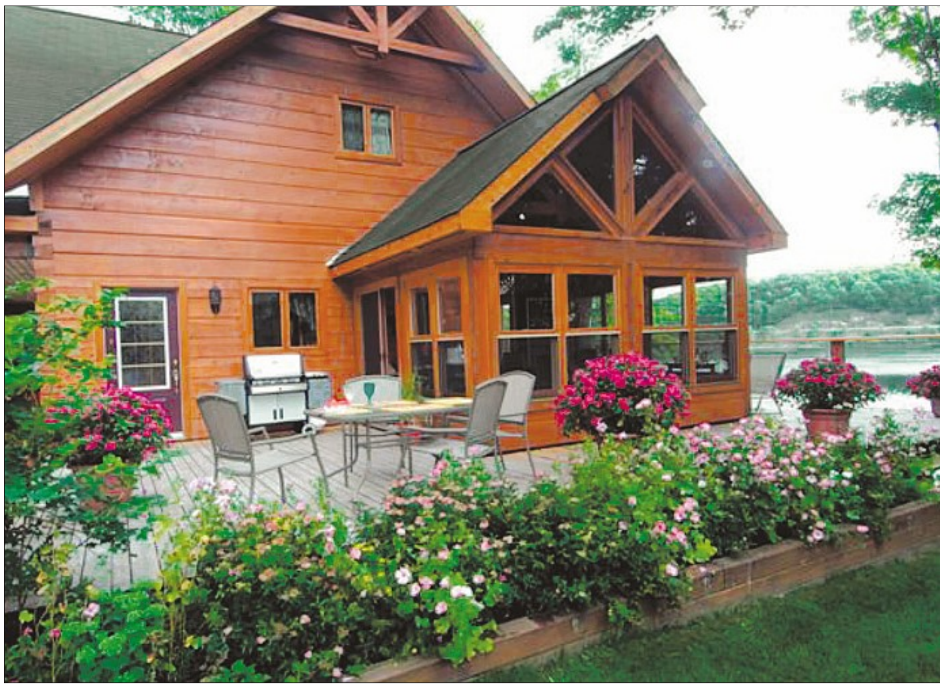
COURTESY 1867 CONFEDERATION LOG HOMES
